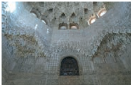
Figure 30. Sala de las Dos Hermanas (Hall of the Two Sisters), Alhambra, Granada, Spain. Built by order of Mohammed V. Ceilings carved in the 16th century (AlhambraDeGranada.org). Photography 18.08.2009 © Joaquim Santos
