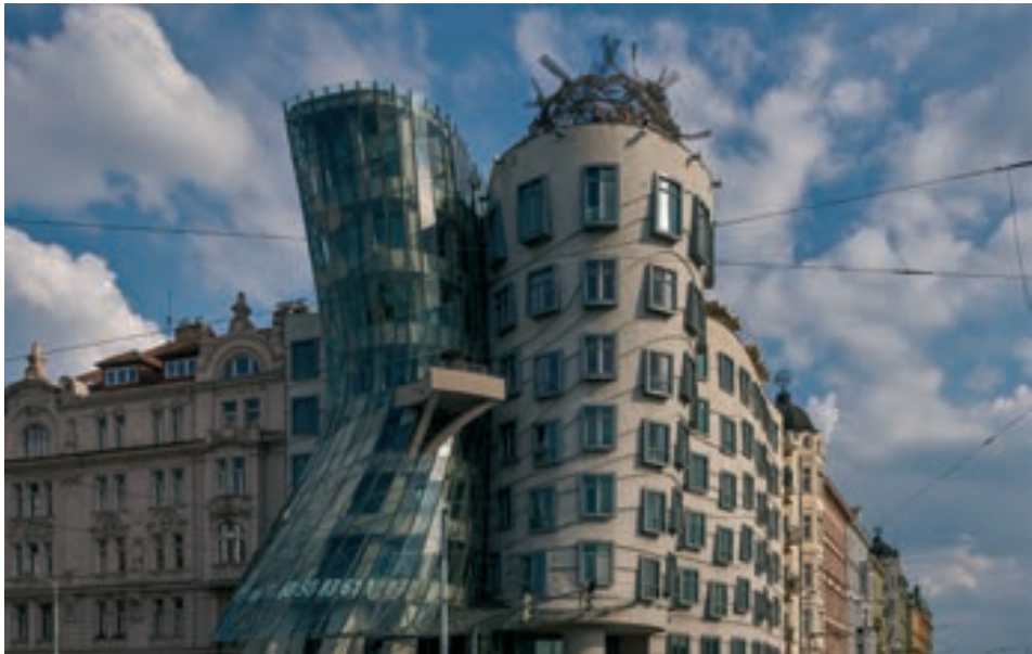
Picture 8 - "Dancing house" by Frank Gehry - Praha
