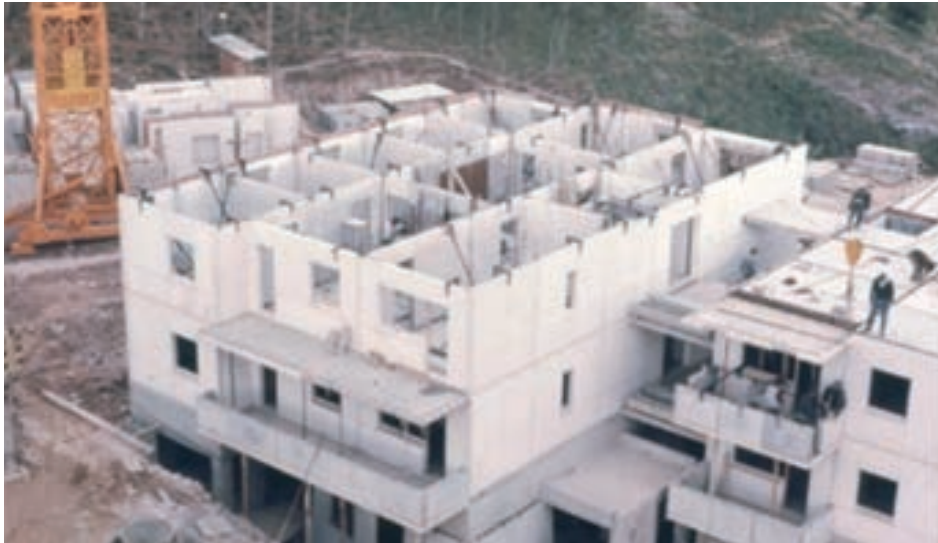
Figure 1 - SAC - Assembly of the panels on site. Source: Reaes Pinto/ICESA 1968
