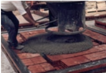
Figure 24 - Concrete Likeage. Source: Reaes Pinto/ICESA 1966
