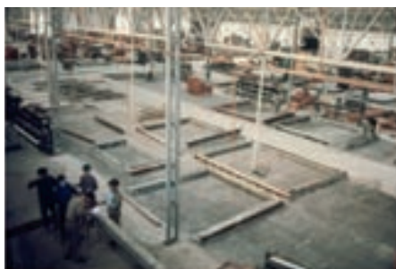
Figure 20 - General view of the factory – metallic horizontal moulds. Source: Reaes Pinto/ICESA
