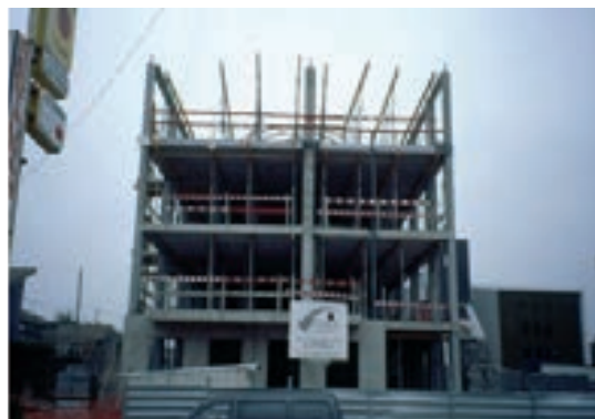
Figure 2 - Partial prefabrication of exterior walls - conventional metallic structure. Souce: Reaes Pinto.
