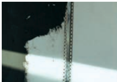
Figure 74 - Building work in progress (Instituto Superior de Ciências Sociais e Políticas – Lisboa) The rendering system is constituted by two layers reinforced with fibreglass mesh. Source: Reaes Pinto, 2000.
