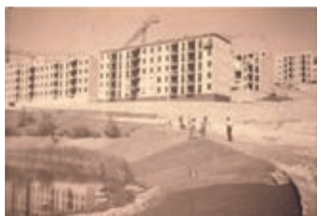
Figure 52 - SAC - Assembly of panels on site. Source: Reaes Pinto/ICESA 1966
