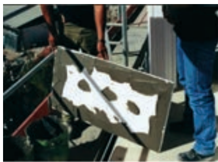
Figura 71 - Building work in progress (Instituto Superior de Ciências Sociais e Políticas - Lisboa) - The insulation boards adhesive coat applied with points and bands. Source: Reaes Pinto, 2000.
