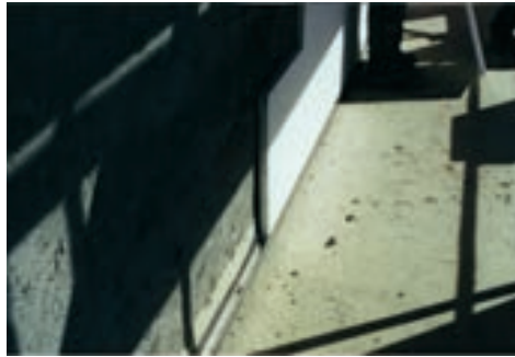
Figura 73 - Building work in progress (Instituto Superior de Ciências Sociais e Políticas – Lisboa) Special fitting profiles to allow an adequate fitting of the pieces and the better continuity. Source: Reaes Pinto, 2000.
