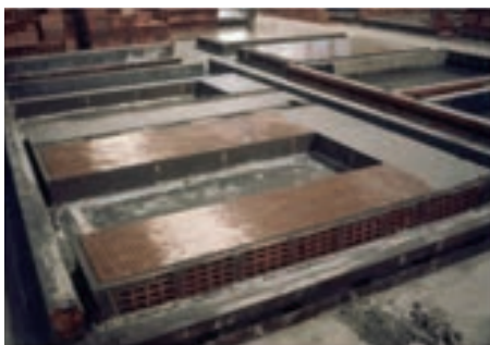
Figure 26 - Resistente Interior Panels. Finishes with ceramic tiles for kitchens. Source: Reaes Pinto/ICESA 1968
