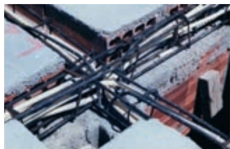
Figure 50 - Network of electric tubes in the reinforced concrete belts, in the panels connections area (previous to the concreting). Source: Reaes Pinto/ICESA 1968
