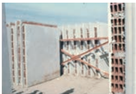
Figure 32 - Regularisation of the concrete layer of the Slab Panel. Source: Reaes Pinto/ICESA 1968
