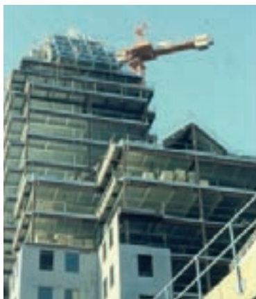
Figure 2 - Partial prefabrication of exterior walls - conventional metallic structure. Souce: Reaes Pinto.
