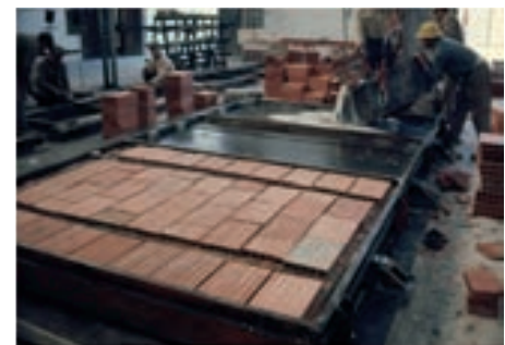
Figure 26 - Resistente Interior Panels. Finishes with ceramic tiles for kitchens. Source: Reaes Pinto/ICESA 1968
