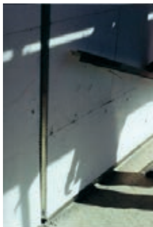
Figura 72 - Building work in progress (Instituto Superior de Ciências Sociais e Políticas - Lisboa) - The insulation boards should be placed in rows with non-continuous vertical joints. Source: Reaes Pinto, 2000.
