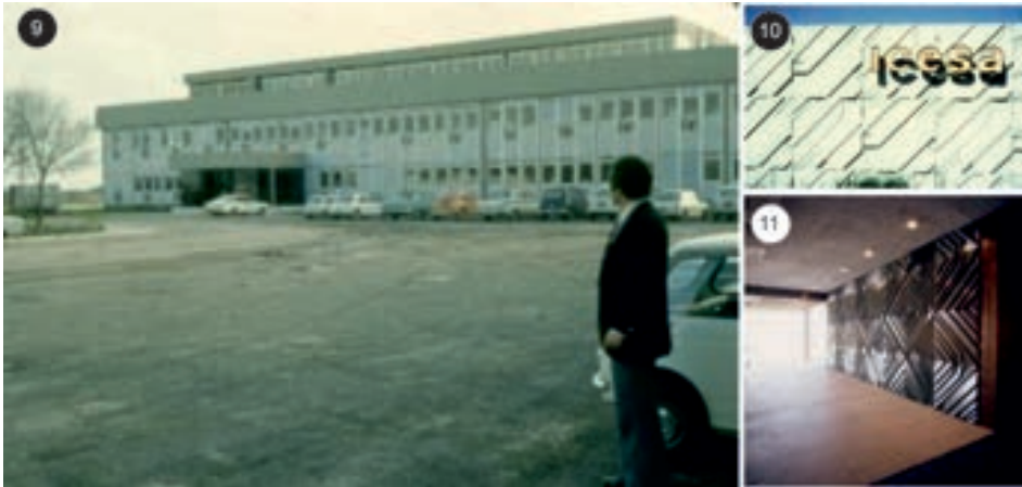
Figure 9 - ICESA Headquarter. Source: Reaes Pinto/ICESA 1971. Figure 10 - Prefabricated decorative panel. Entrance to the company complex. Source: Reaes Pinto/ICESA. Figure 11 - ICESA Headquarter entrance. Source: Reaes Pinto/ICESA 1972.
