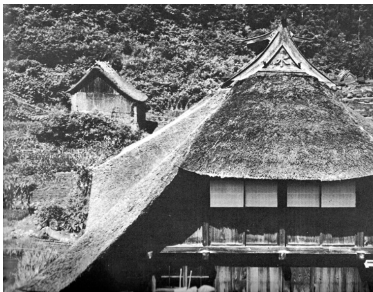
Ilustração 9 – “Vegetal Roofs”, Japan. (Architecture Without Architects, RUDOLFSKY, imp. 1964, im.145)
