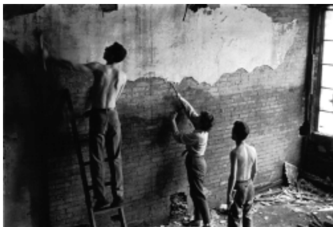
Ilustração 25 – Residents Exposing Brick Wall in Loft, Broome Street, SoHo. Dorothy Koppelman, 1963. (Dienes, s.d.).
